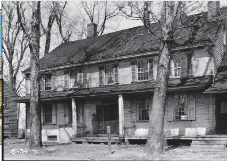
Fig. 4: A photo from the Historic American Buildings (HABS) collection, NJ-134 showing the Lawrie House ca. 1933. 3
