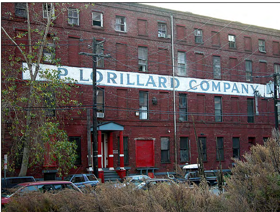
Fig. 7: A 2007 view of 111 First Street shortly before demolition to make way for a luxury condo high rise. 3
