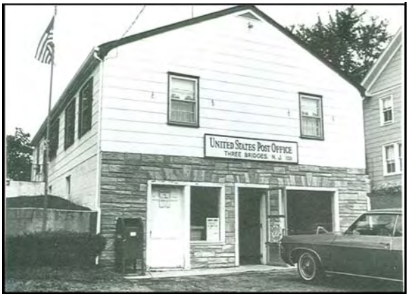
Fig. 152: Another location, since replaced.
