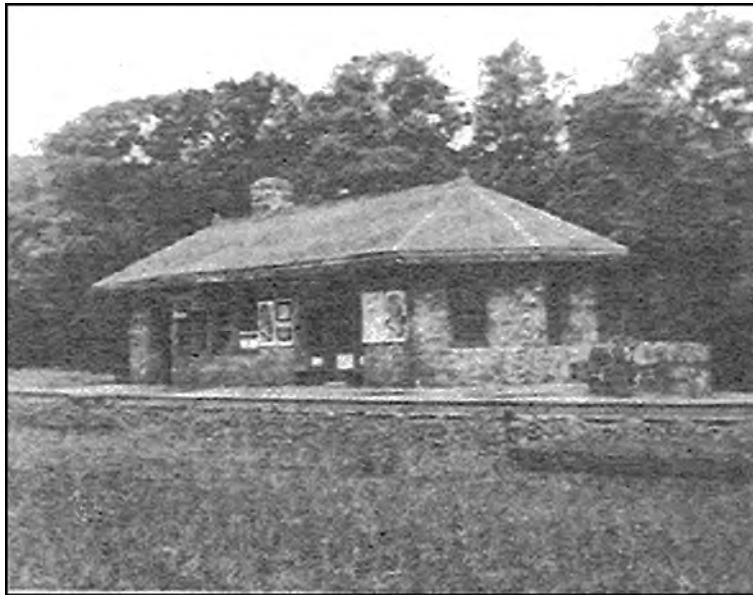
Fig. 8: The Central Railroad Station at Ludlow formerly known as Asbury Station.
