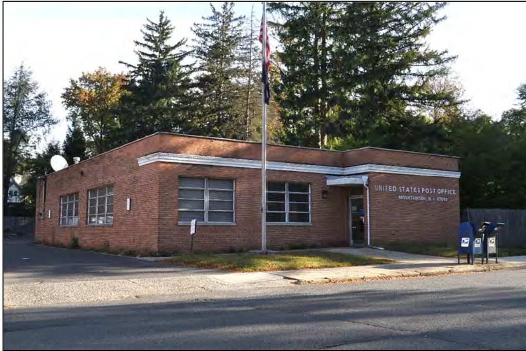
Fig. 11: Current photo of the Mountainside Post Office, 604 Sherwood Parkway.
