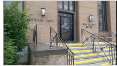
Fig. 12 & 13: View of Ocean City PO in construction in 1937, and as it appeared in 2016.
