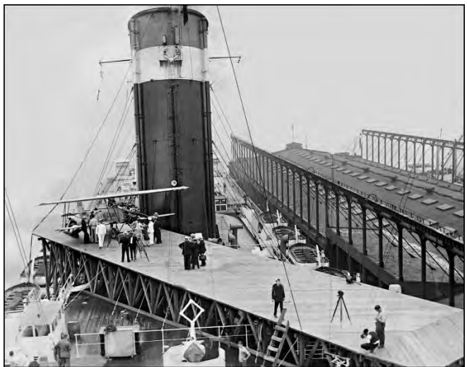
Fig. 5: Showing the runway built of wood which was added to the deck of the Leviathan.
