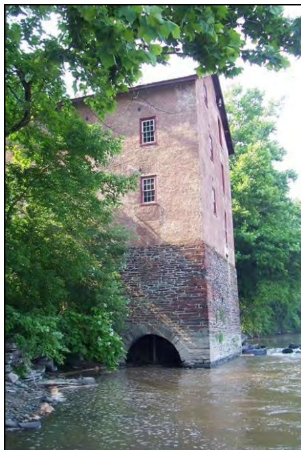
Fig. 9: Stover Mill, river view.
