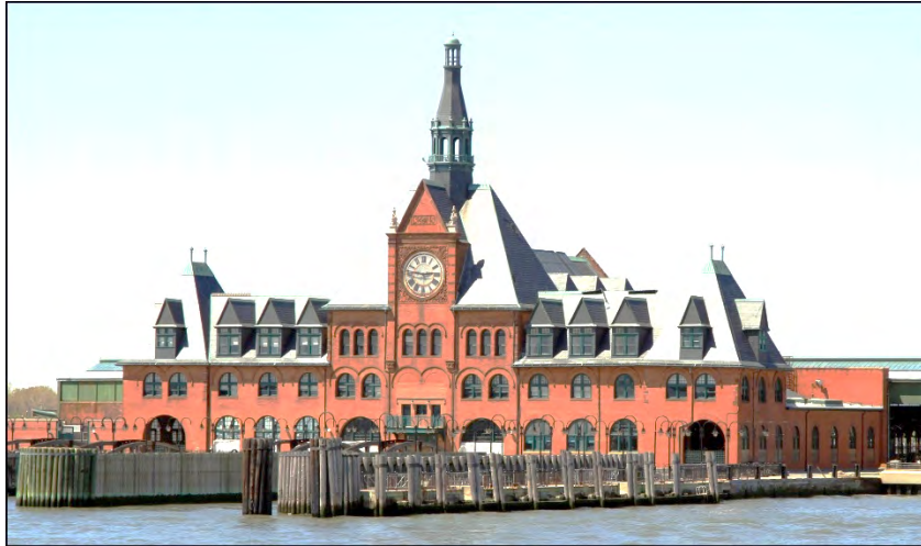
Fig. 15: Compare with Fig. 10 above. This last vestige of the railroads in Jersey City, the Central RR Terminal, viewed today, now serves as the terminal for ferries to Liberty & Ellis Islands from the Jersey side of NY harbor. 2
