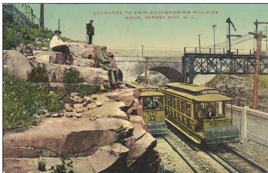
Fig. 2: Approaches to Jersey City through and around the end of the Palisades, using both tunnels and cuts.
