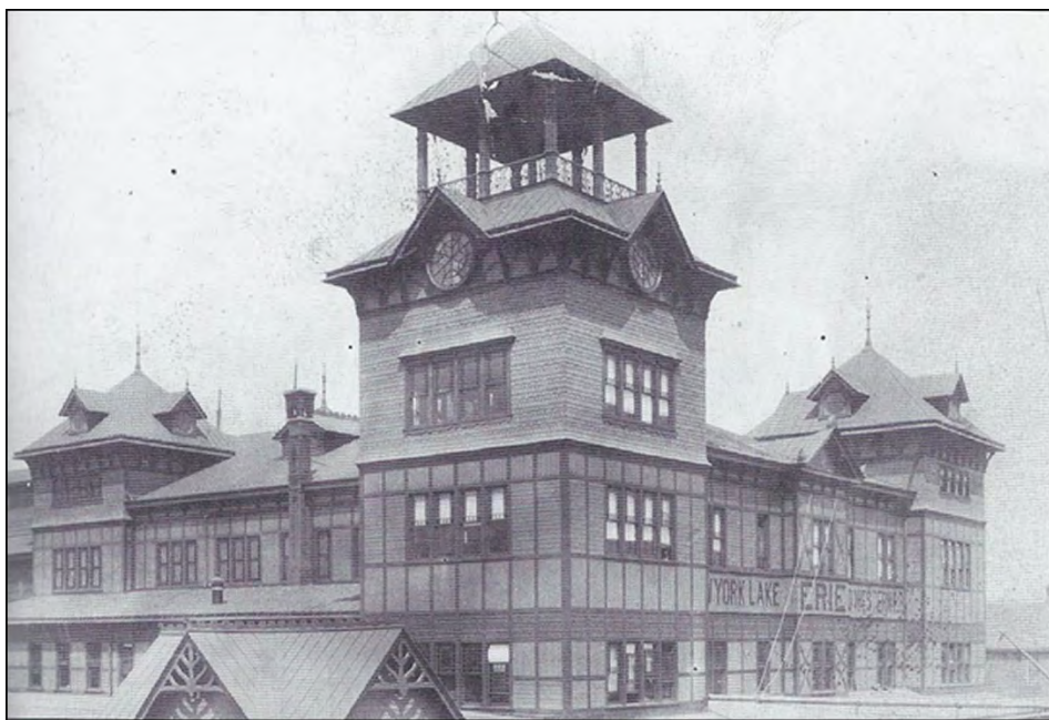
Fig. 14: The Erie Terminal at the foot of present day Pavonia Avenue. Note the proper name of the line across the front of the building, New York, Lake Erie & Western Railroad.
