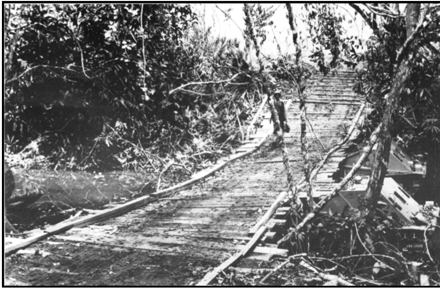
Fig. 10: The makeshift bridge constructed using two amphibious vehicles (LTVs or "amtracs" for support in the middle. These vehicles were very useful for beach landings of men and materials (and improvising bridges), but they lacked armor for protection when landing under fire.
