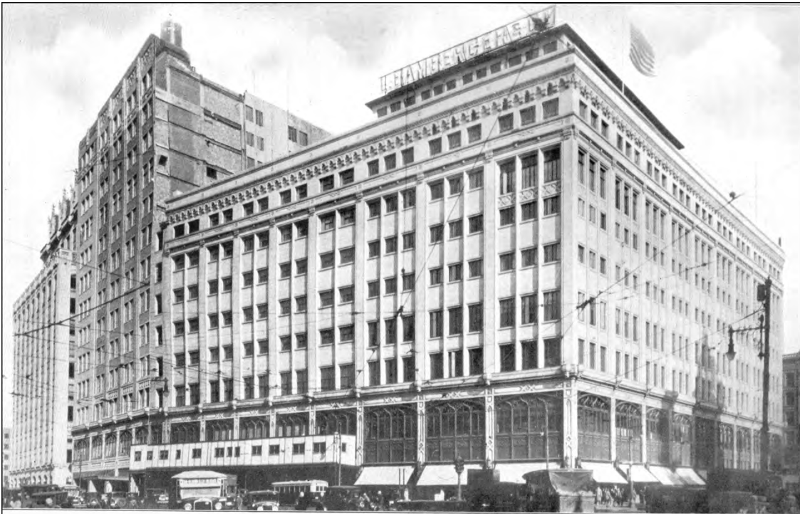
Fig. 1: Bamberger's Department Store occupying an entire block in Newark between Market, Washington, Bank, and Halsey Streets.
