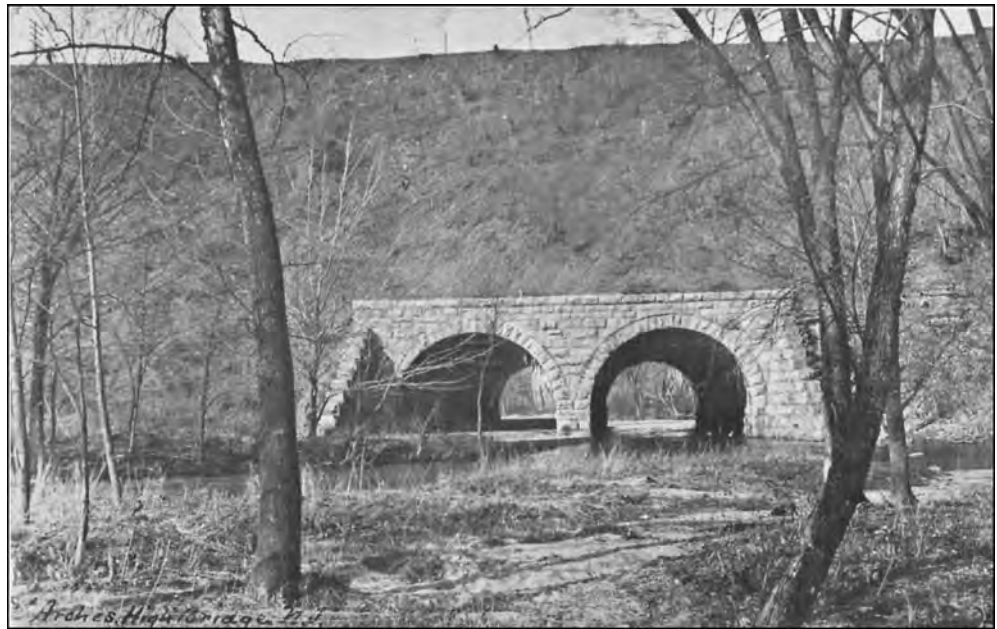
Fig. 4: A post card view of The Arches created to carry the river (on the right), and the road (on the left), beneath the embankment built over the bridge. They are (of course) on Arch Street in High Bridge
